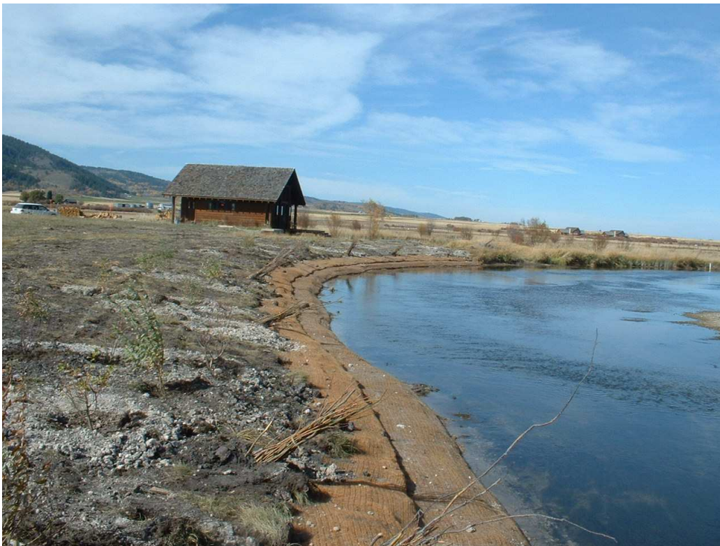
Willows and Soil Lifts Installed (October 2002).
